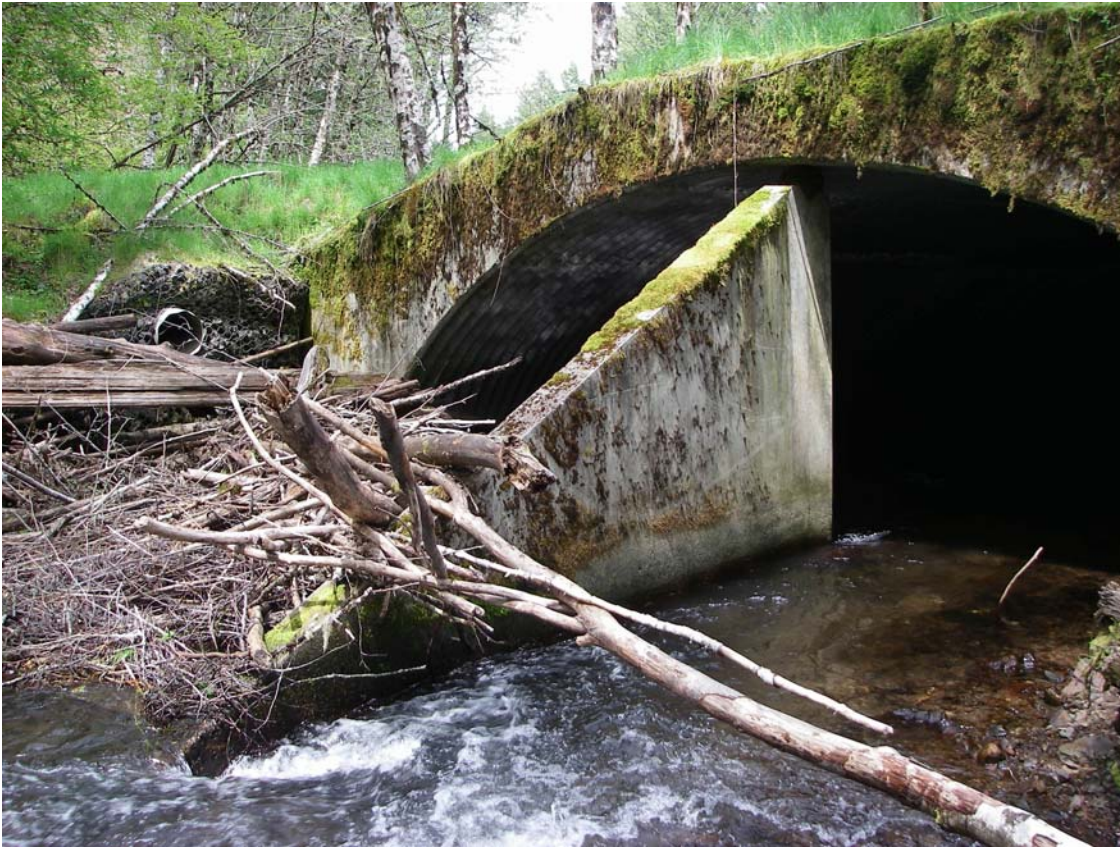
Photo 6. Hwy 26 culvert SF Rock.
