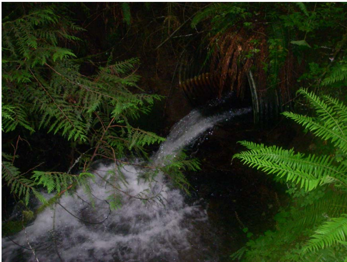
Photo 19. Culvert in Trib A of Selder Cr.
