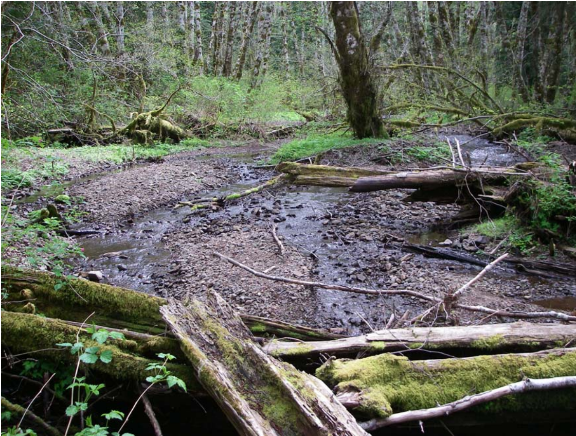
Photo 7. Area treated with full spanning wood jams, Anchor Site 2 in SF Rock.
